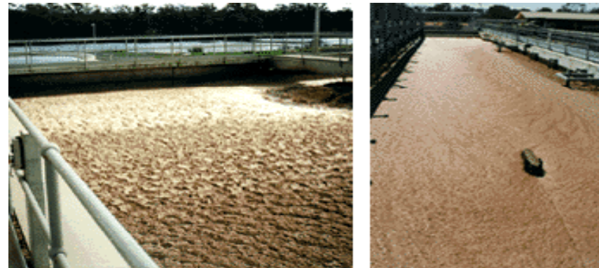
Figure 1. Foaming in two Australian activated sludge plants. Plant on right is an oxidation ditch with foam covering the dividing wall.
